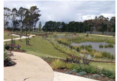
Constructed wetlands emulate the water filtration functions of natural wetlands, and can also create useful habitat.
