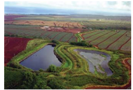
Constructed ponds help clean the water supply and reduce downstream erosion and flooding.
